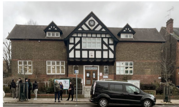
Mock Tudor Facade.
