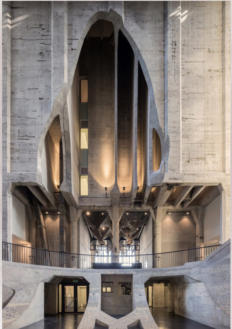
Fig. 2 - the majestic entrance hall revealing the cut through the vertical tubes
