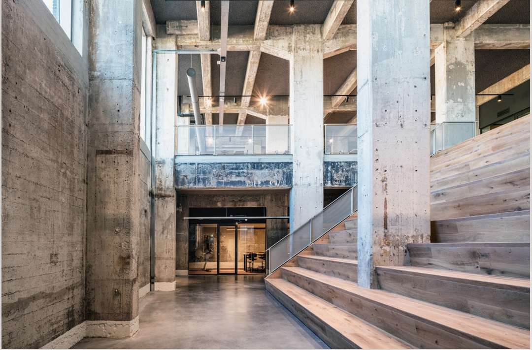
Fig.17 - retained original skeleton of the building and its aged texture
