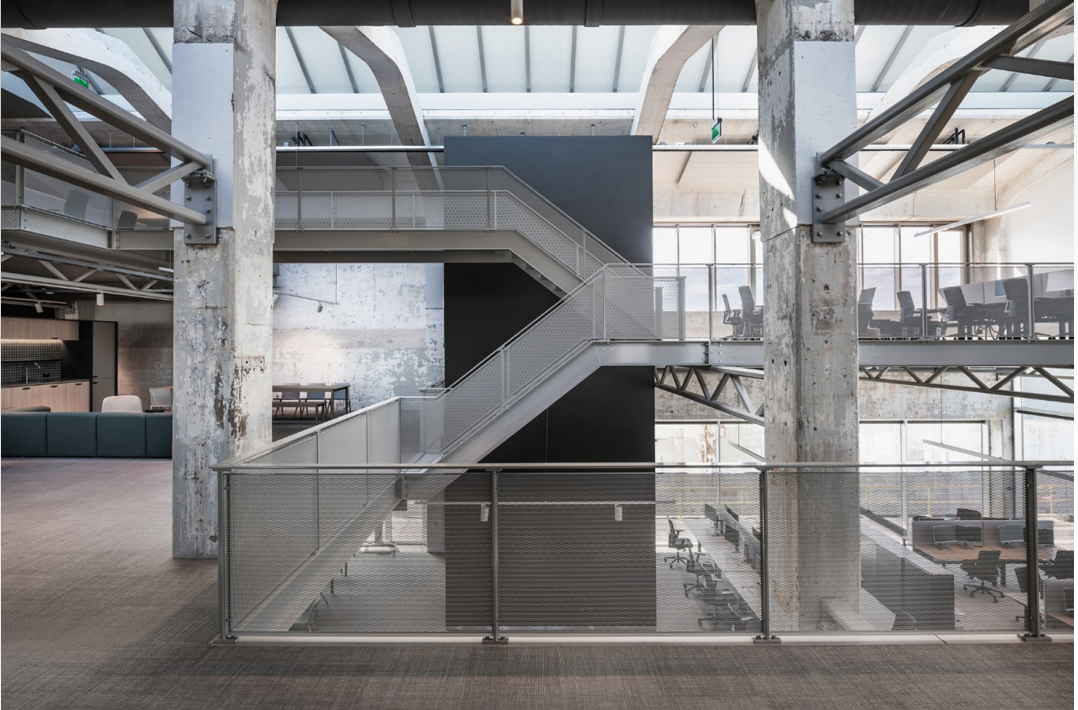
Figure 20 - levels and steel construction
