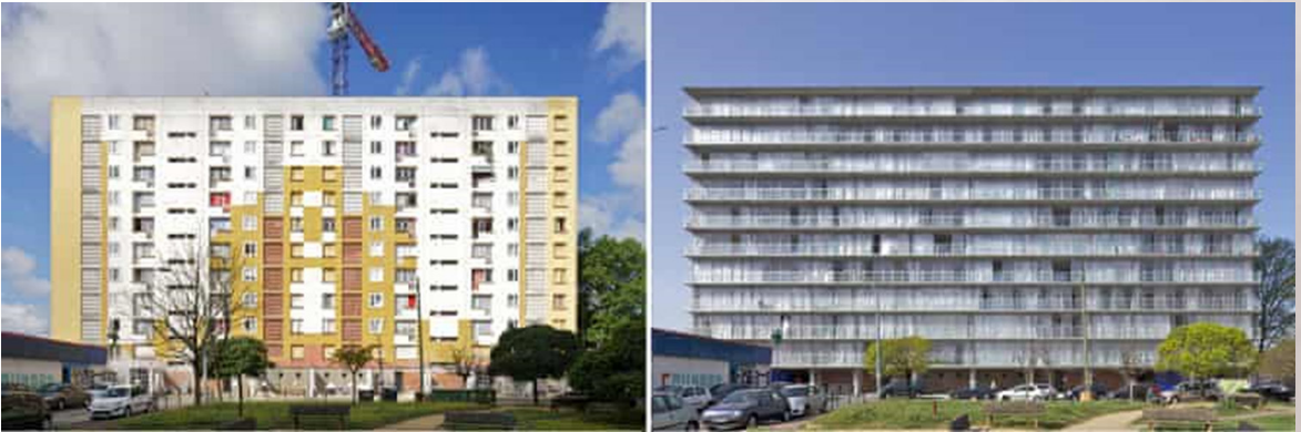
Fig.8 - Before and after the transformation of Grand Parc, Bourdeaux by Philippe Ruault
