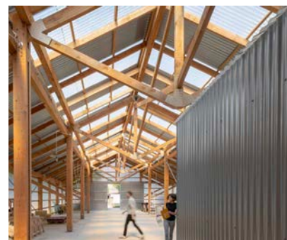
Fig.4: Interior of the space, exposed timber frames
