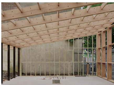
Figure 9 Feilden Fowles' studio in south London uses lengths of UK-grown Douglas fir in a simple pitched extrusion
