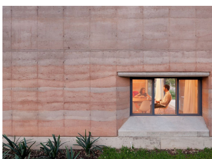
Figure 11 Tatiana Bilbao architects use rammed earth to construct an adaptable, vernacular house in Jalisco
