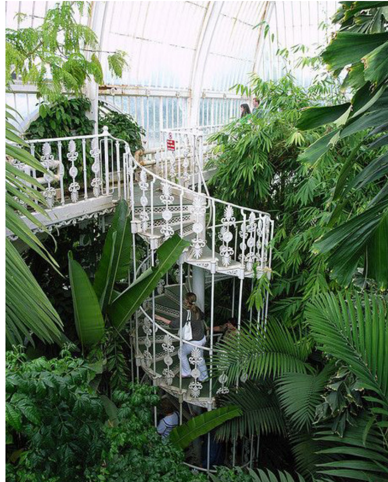
Figure 11. wrought iron structure (Cadman, S. (2008))
