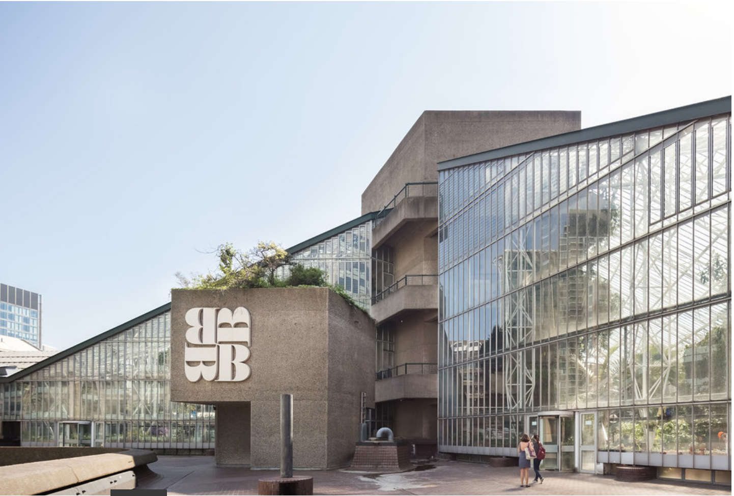
Figure 12. The Conservatory on the roof of the Barbican Centre (Bradley, D. (2018))
