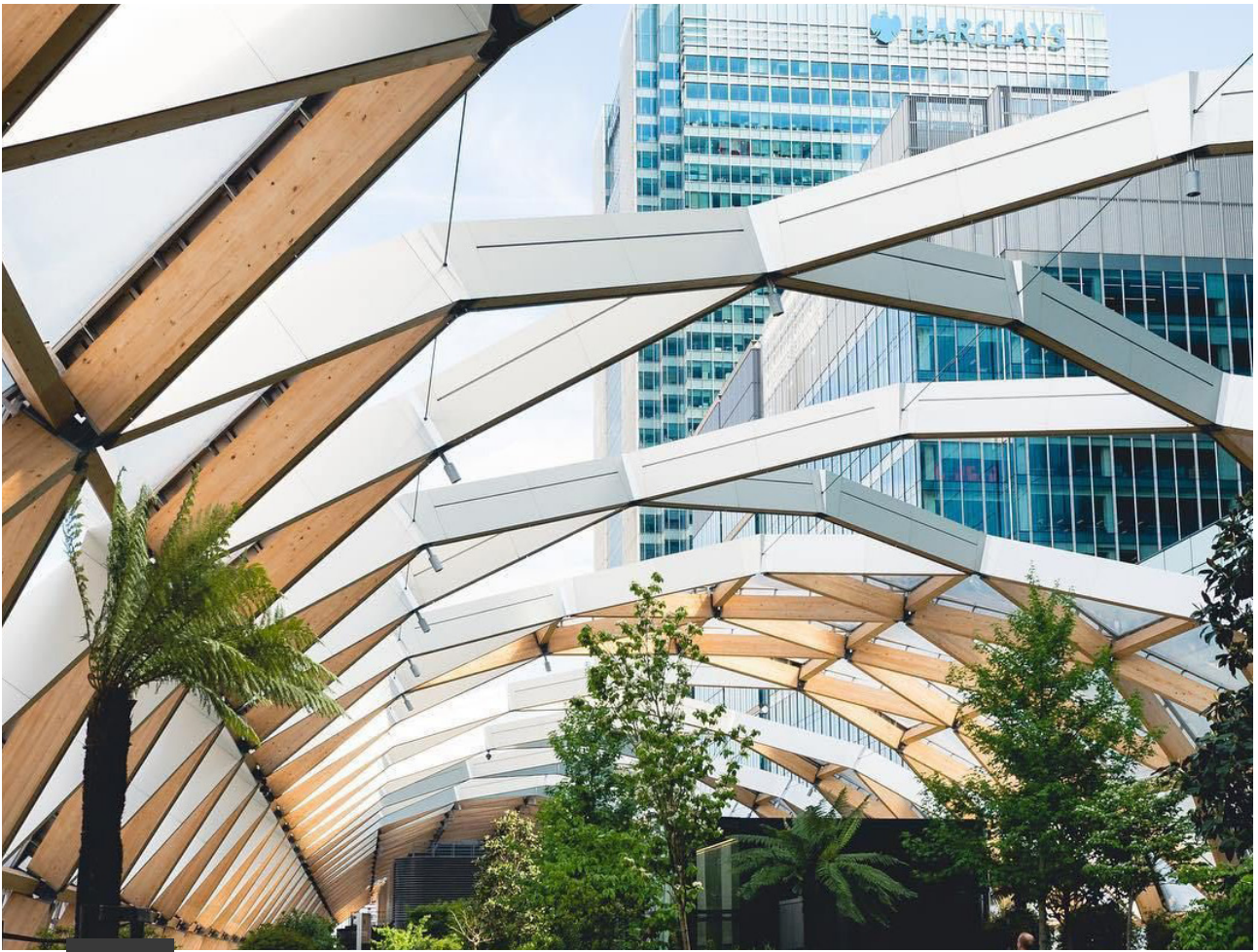
Figure 30. ETFE roof at Roof garden, Canary Wharf Crossrail Station, Crossrail Place (Lee, 2015)
