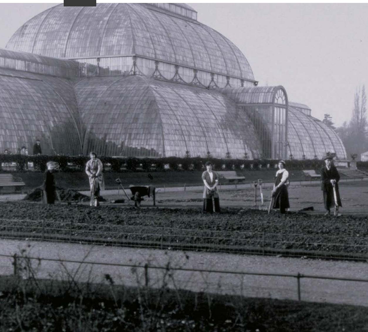
Figure 21. Workers outside the Palm House (Gardens, 1857)
