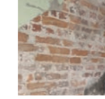
Exposed 17th Century Existing Brickwork
