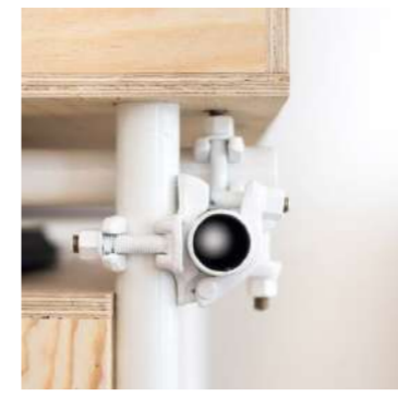
recycled scaffolding used for the whole interior structure
