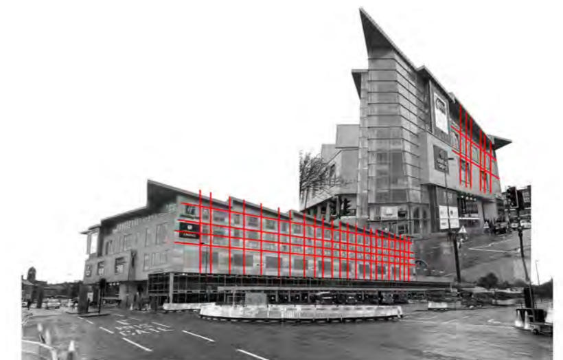
Fig. 98. Diagram of Derby Coach Station Holiday Inn where 200 +/- refugees reside for months due to government policy confined to their rooms (Newens,G.,2024).
