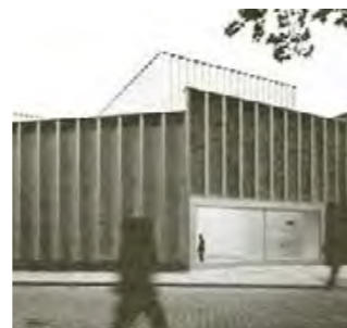
Fig 66. Nottingham Contemporary art gallery, designed by Caruso St John Architects (Caruso St John, n.d.)
