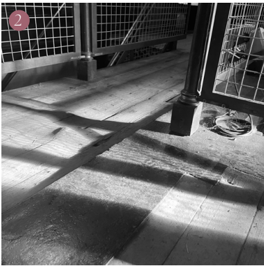
Warped Wooden Floorboards (First Floor, Engine House): The warped boards express time and wear. These have been retained or reused elsewhere in the scheme rather than being discarded.
