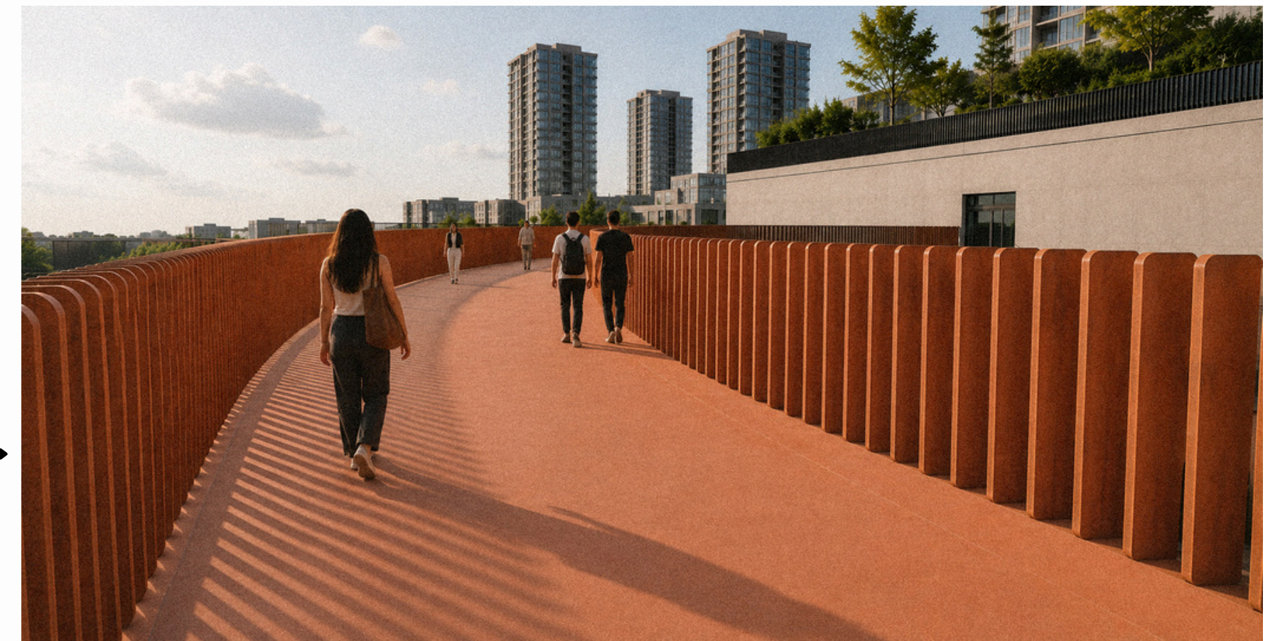
Elevated pedestrian bridge
