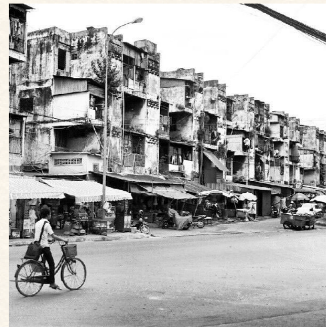
Figure B.04. Deteriorating White Building.
