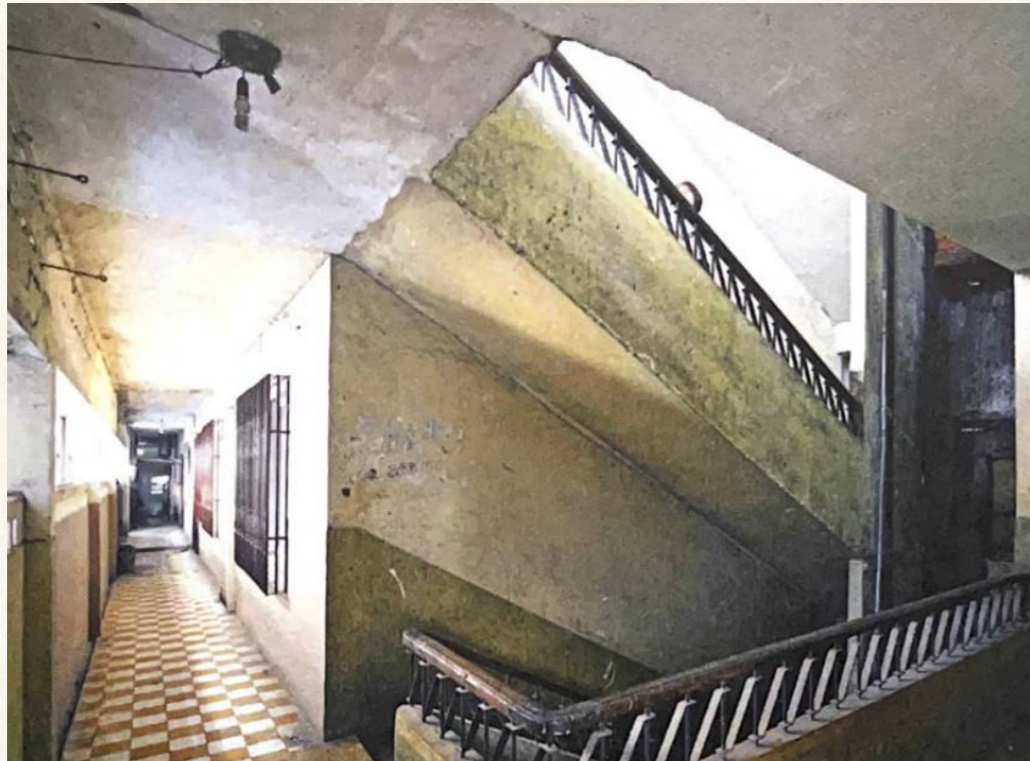
Figure 28. Shared main staircase
