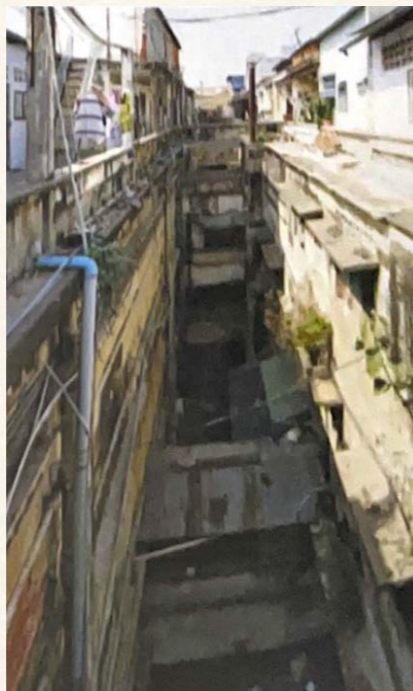
Figure 26. Shared courtyard condition
