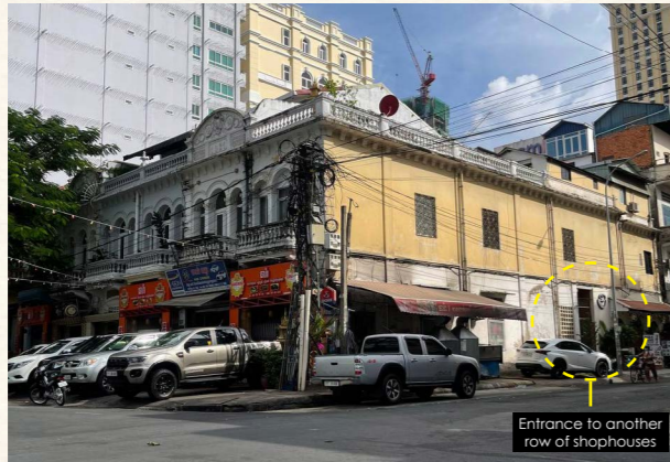
Figure 23. Corner view of shophouses on Street 108 and Street 53
