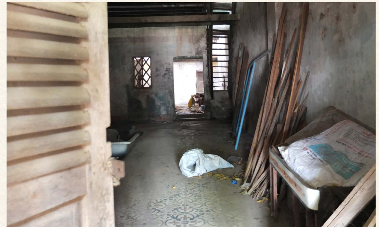
Figure 47 Site survey photo of existing encaustic tiles before renovation.
