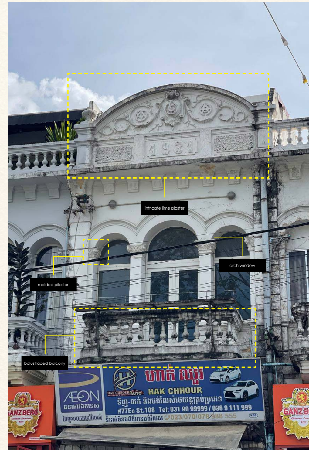
Figure 22. Close up of the most elaborate facade
