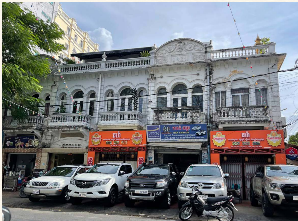
Figure 21. Intricate facade of row of shophouses on street 108
