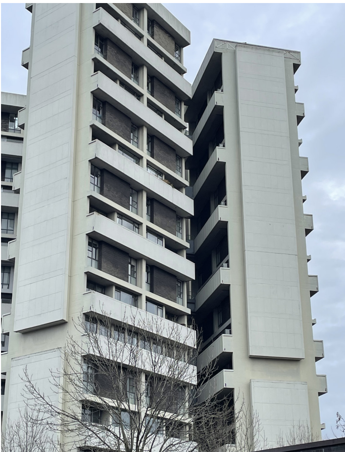
Figure 7: Primary Photograph– Right facade 01/2022
