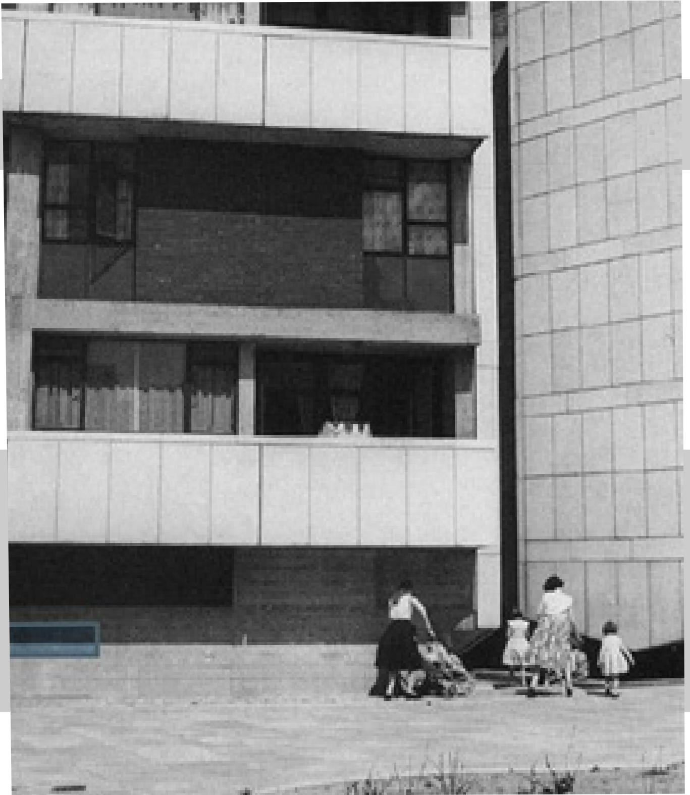
Figure 10: Residents onsite- Ground floor Maisonettes
