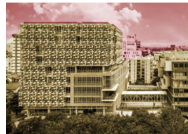
Figure 15 - External view of Project legacy, edited by Camila Zuniga (William McDonough + Partners, 2021)
