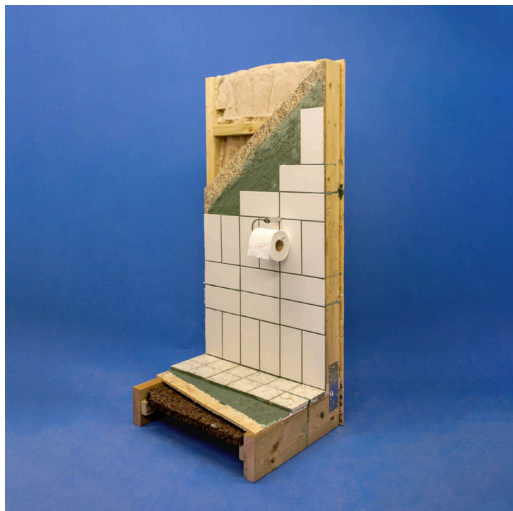
Figure 9 - Wall build up prototype, made by Material Cultures in collaboration with After School Club and Store Projects (Material Cultures, 2023)
