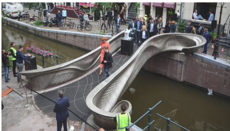
fig 2.10 3D-printed steel bridge in Amsterdam
