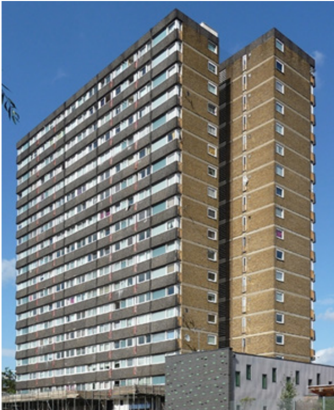
fig 2.2 Agar Grove Estate, Camden is an example of a typical council block in United Kingdom
