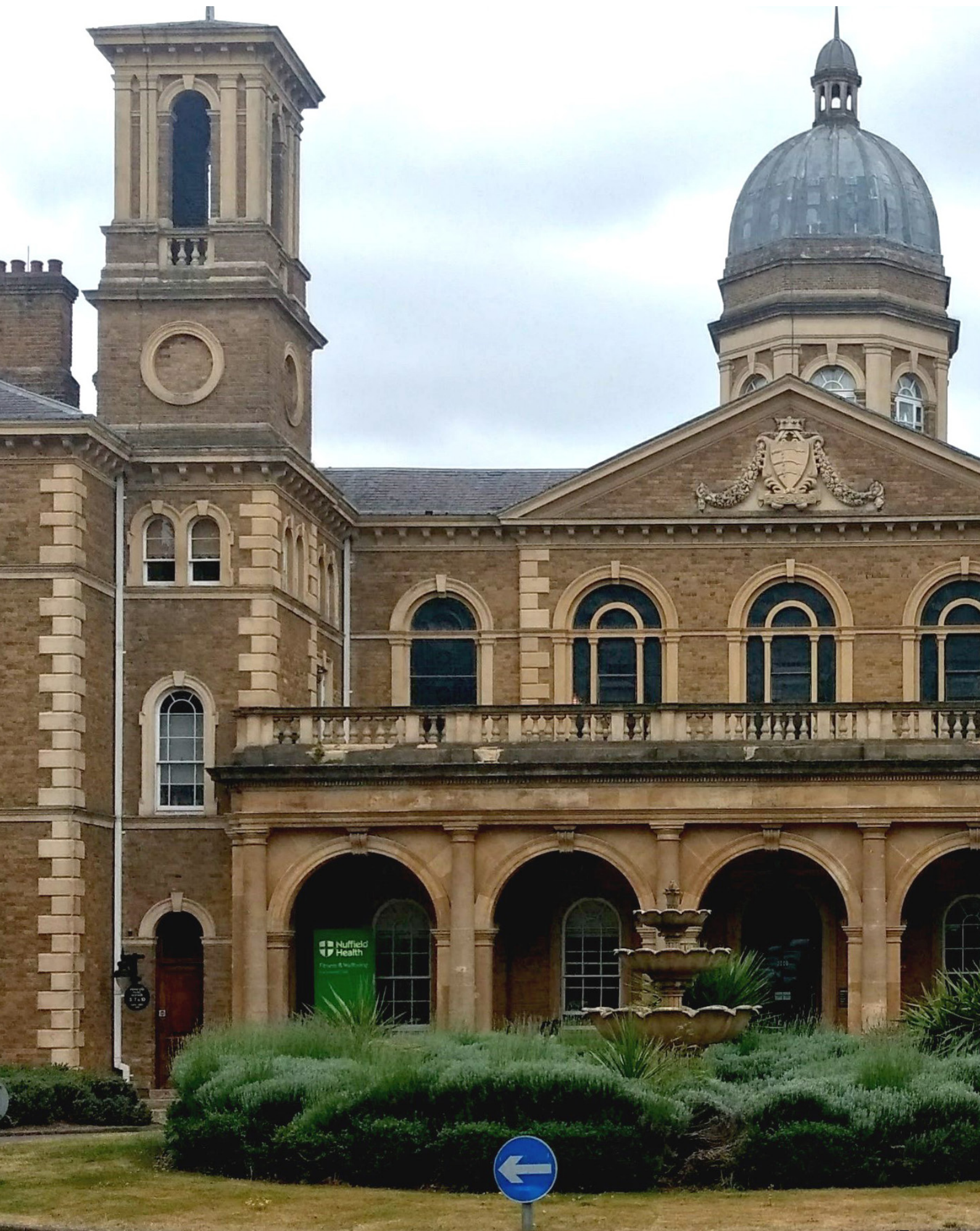
Figure 31: Princess Park Manor
