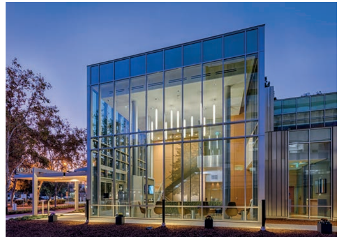
Figure 21: The Exterior of the Taube Pavilion
