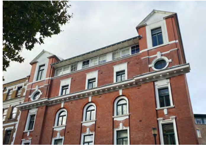
EXTERIOR OF BUILDING
