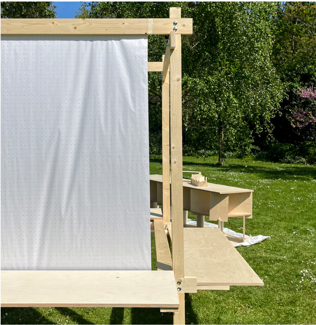
Detail 02: Stacked lap joints use m12 bolts tightening under strain eliminating the use of epoxy or nails a technique optimised for reuse.
