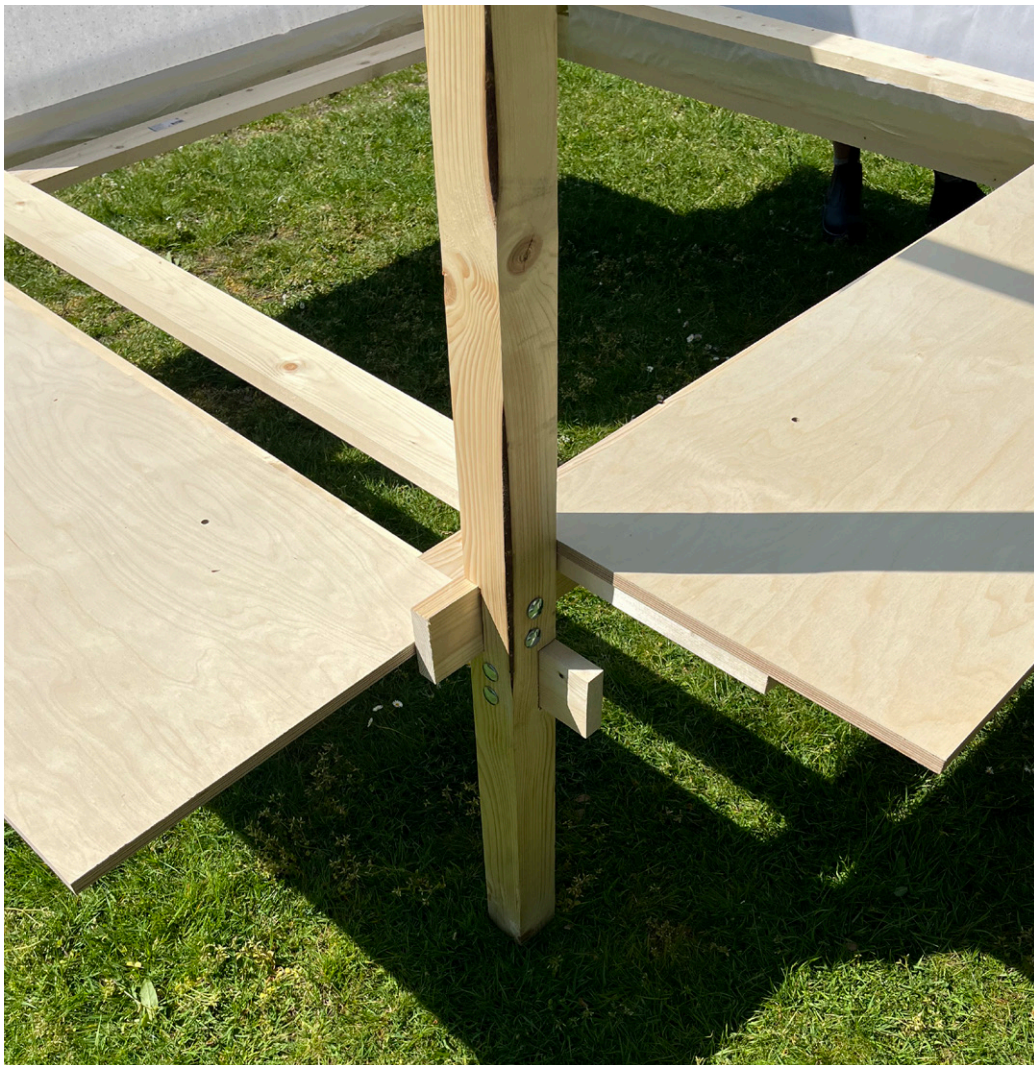
Detail 03: Model surfaces in 18mm fair faced birch plywood are left untreated suitable for future reuse.
