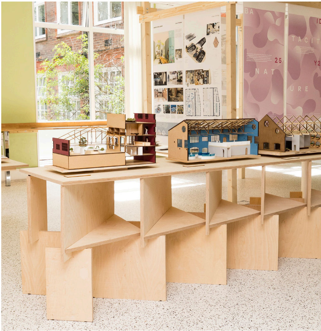
03. The exhibition tables compliment the graphic display architecture, employing the same structural logic. An adapted lap joint allows demounting and reassembly.
