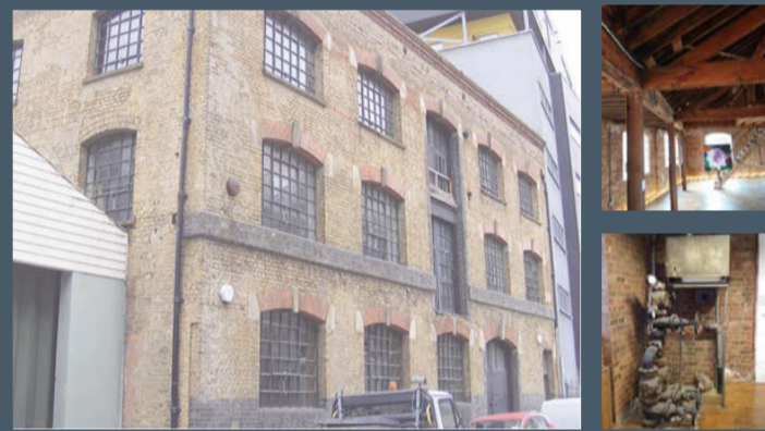
The site is situated in a densely populated area, nestled between a busy road and a major railway. The air quality is poor, and there is high sound pollution, resembling the typical conditions found in London.
