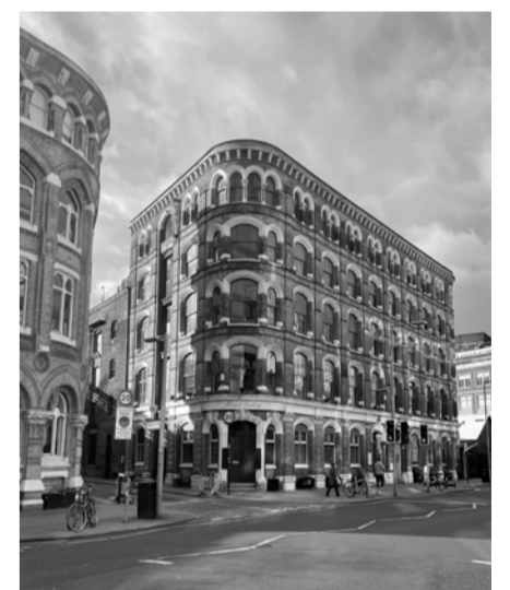
Site - Building's facade
