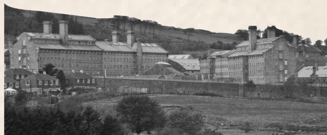
HM Prison Dartmoor operated for over 200 years, this proposal retains the historic boundary walls, while transforming the site into a space centred on rehabilitation.
