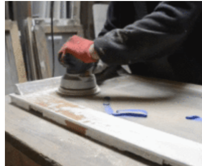
Figure 53. Image showing the wood being sanded down ready for protective treatment. (Critical Concrete, 2020.)
