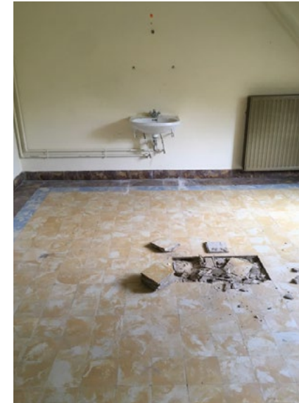
Figure 30. Image showing the removal of Tiles from an unused building by Rotor DC. (Rotor DC, Date Unknown)
