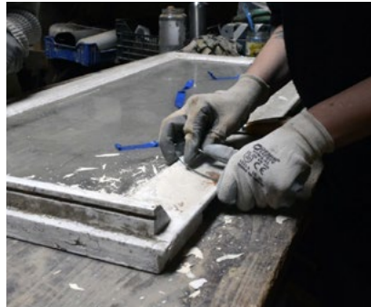
Figure 52. Image showing the process of cleaning the wood using broken glass to scrape off old paint. (Critical Concrete, 2020).
