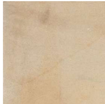
ORIGINAL FEATURE SANDSTONE
