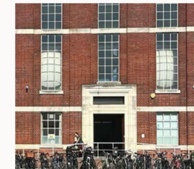
Historic brick facade preserved
