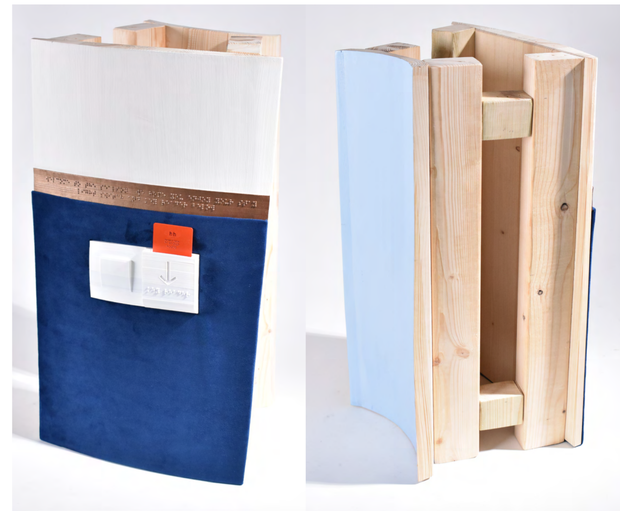
Final model. A section of the Sealion wall has been recreated at a scale 1:1. It shows a light switch and card/key reader next to the main entrance. This real-size model shows how contrast and texture are important for visually impaired users. The EU-style light switch is bigger than the UK ones, making it easier to operate. 1000mm of the bottom part of the walls is upholstered in marine blue velvet by UK Fabrics Online (45,000+ Martindale Rub Score). The velvet wraps the space in one direction, helping to inform the user where they are going based on the pile orientation.
