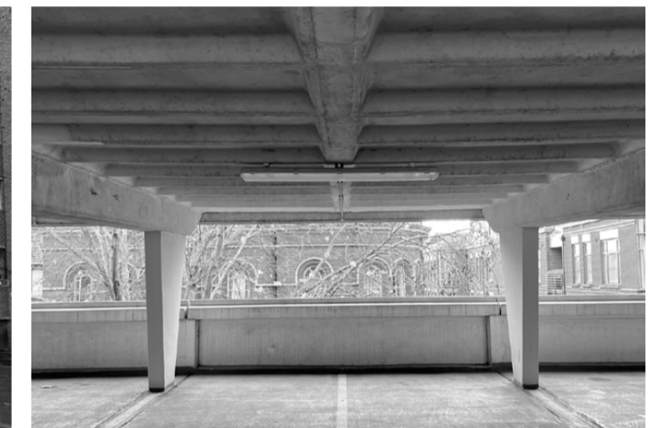
// REINFORCED CONCRETE JOIST SLABS, BEAMS AND COLUMNS PROVIDE DURABLE STRUCTURE, BUT ARE HOSTILE TO ECO-SOCIAL LIVEABILITY.
