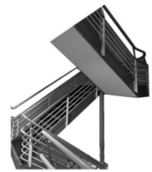
Listed Staircases verticality and materiality
