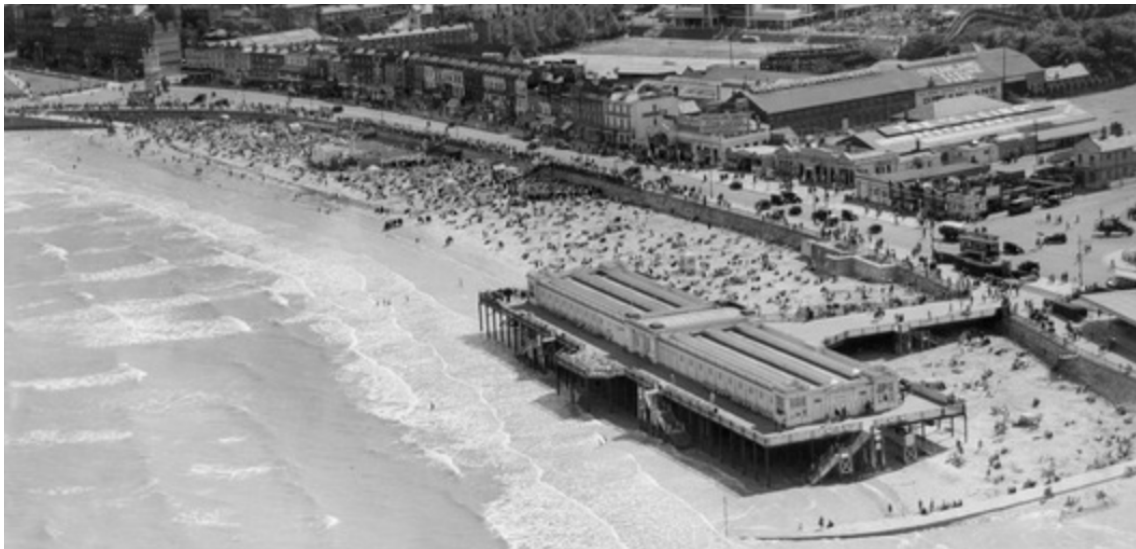
Fig. 16. Overhead shot of Margate's Marine Bathing Pavilion (1933)
