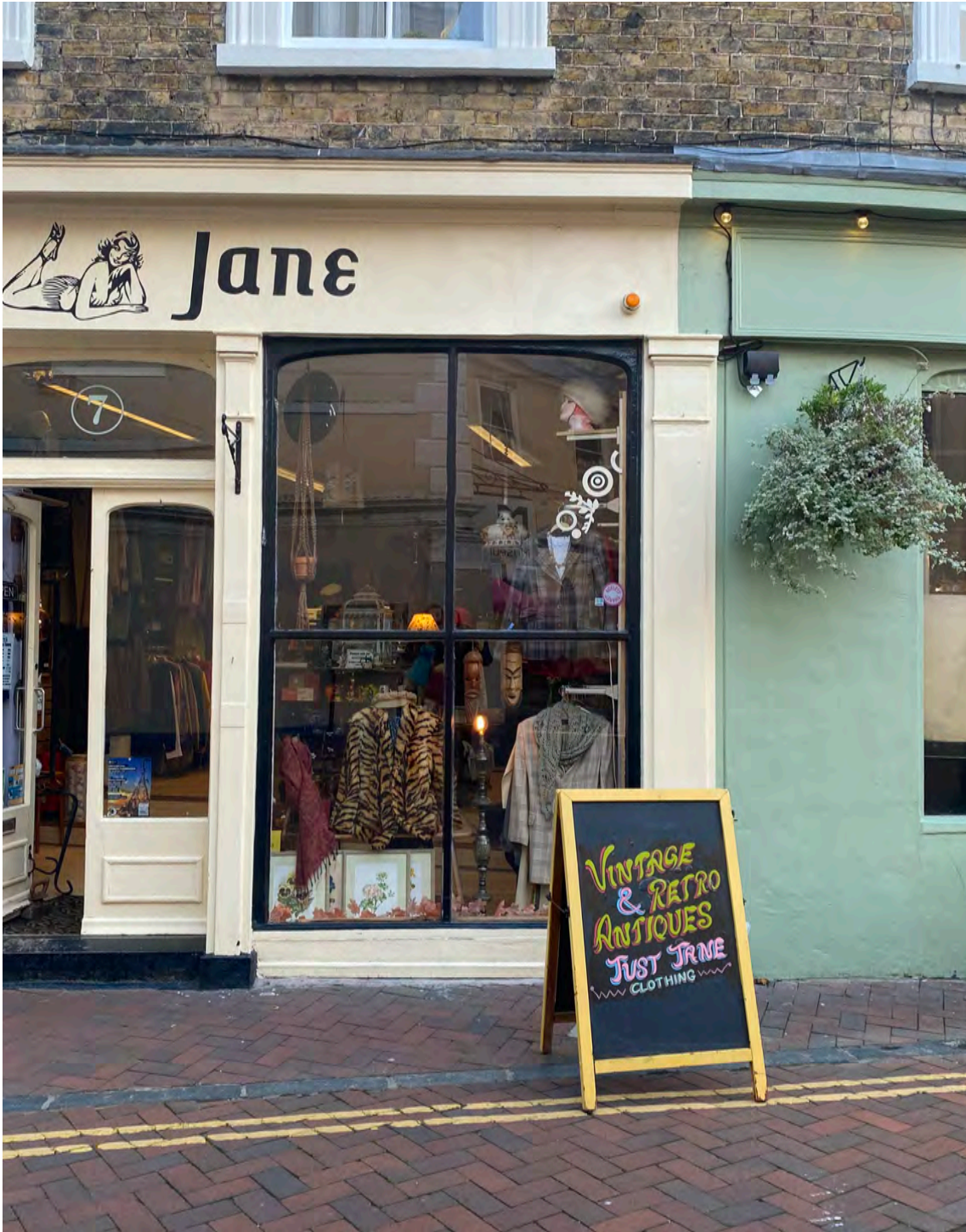
Fig. 31. The Old Town shop front (2023)
