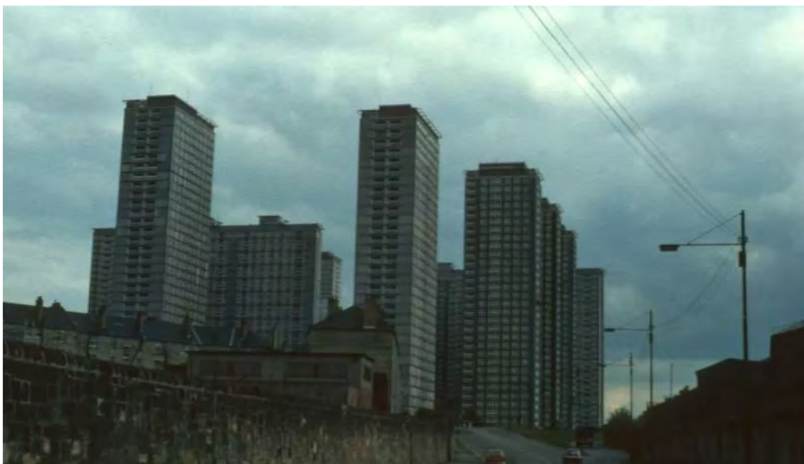
Fig. 2. Glasgow multi-storey red road flats (2022)
