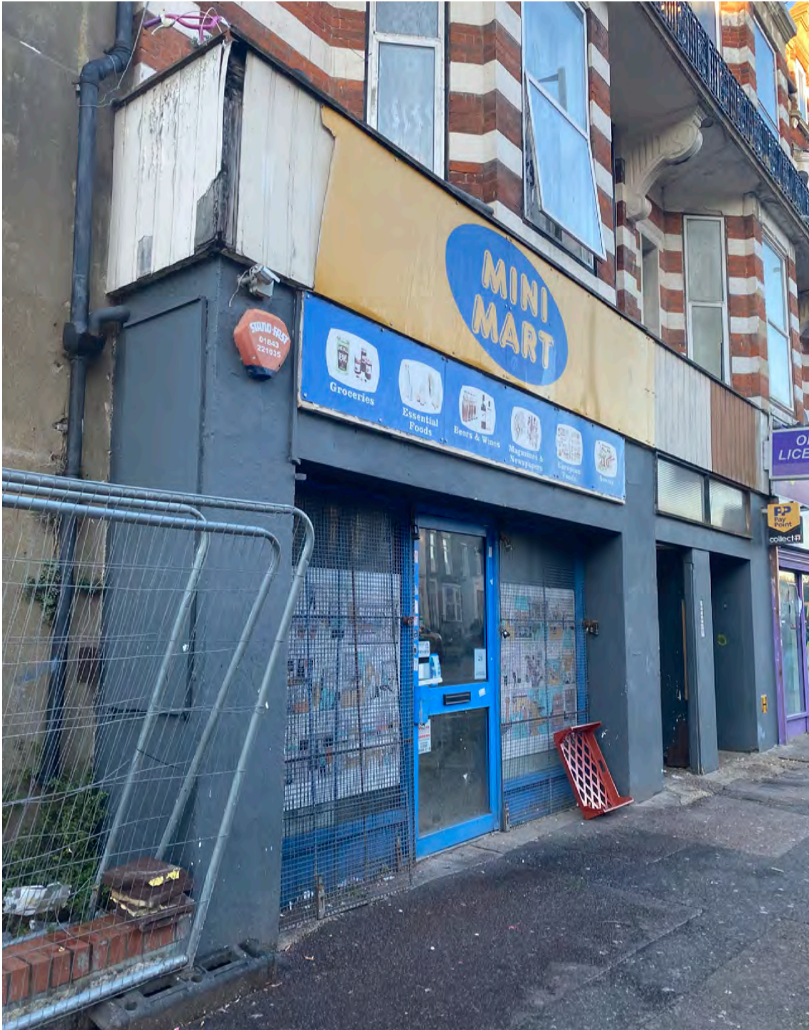
Fig. 26. Cliftonville shop front (2023)
