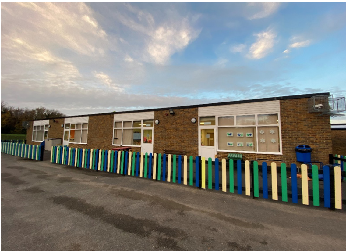
Fig. 4 Satellite school building (2023)
