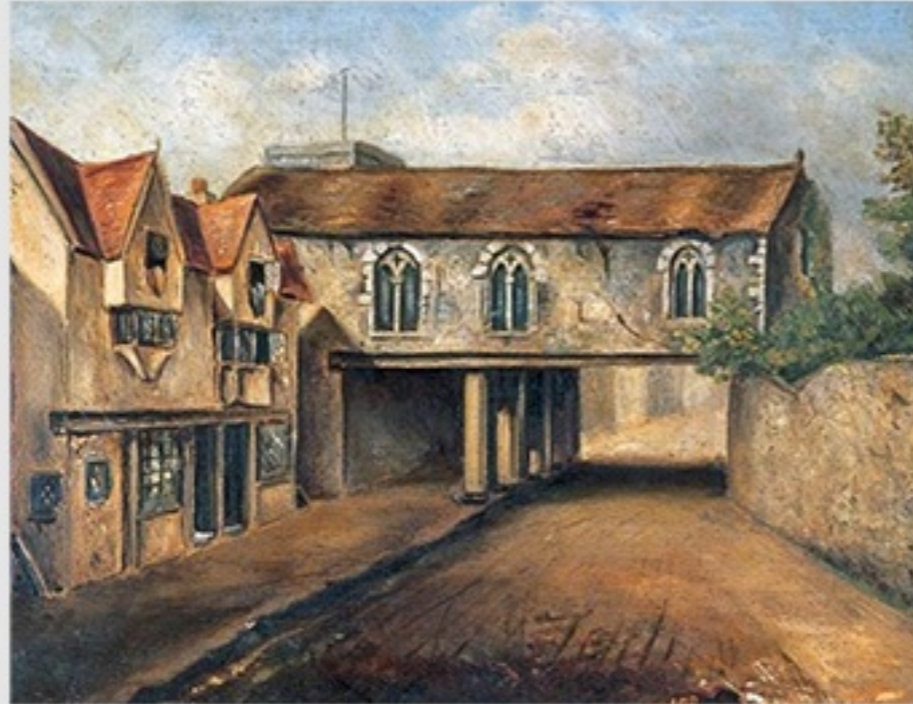
St Mary's church built over Borough street, re-built to allow built to allow horse & larger carriages to go through.
