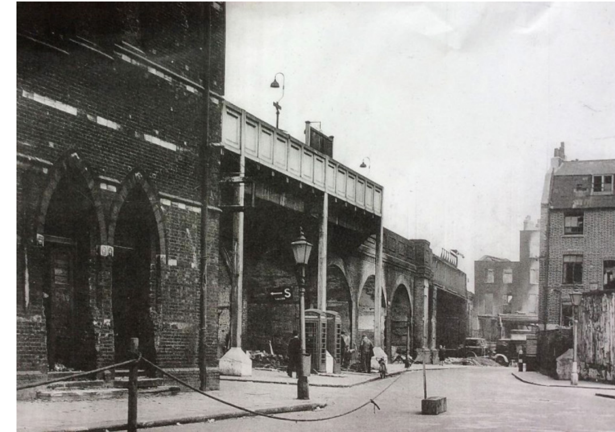
Figure 5- Victorian Railway Arches located on Elephant Road, 1940
