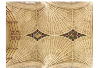
Figure 15: Stone fan vaulted ceiling
