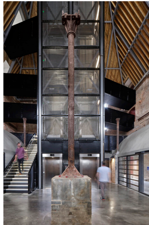
Figure 11: Interior of the flax mill after regeneration, displaying the cast iron column
