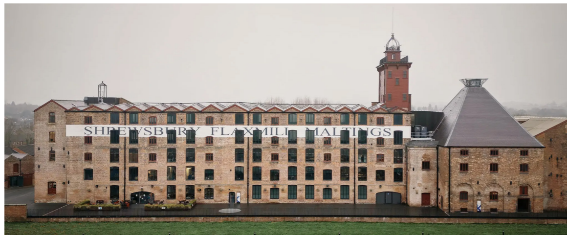
Figure 12: Exterior of the flax mill after regeneration.
