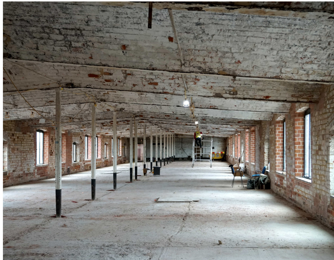
Figure 9: Flax Mill before retrofit
