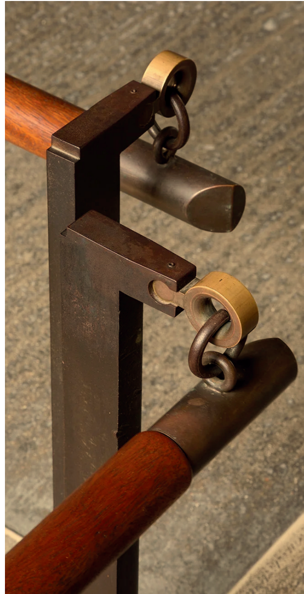
Figure 9 : Bronze pivot hinge at the Castelvechio Museum, illustrating Scarpa's principle of abutment, where new material meets historic fabric through precise articulation rather than material merging.
