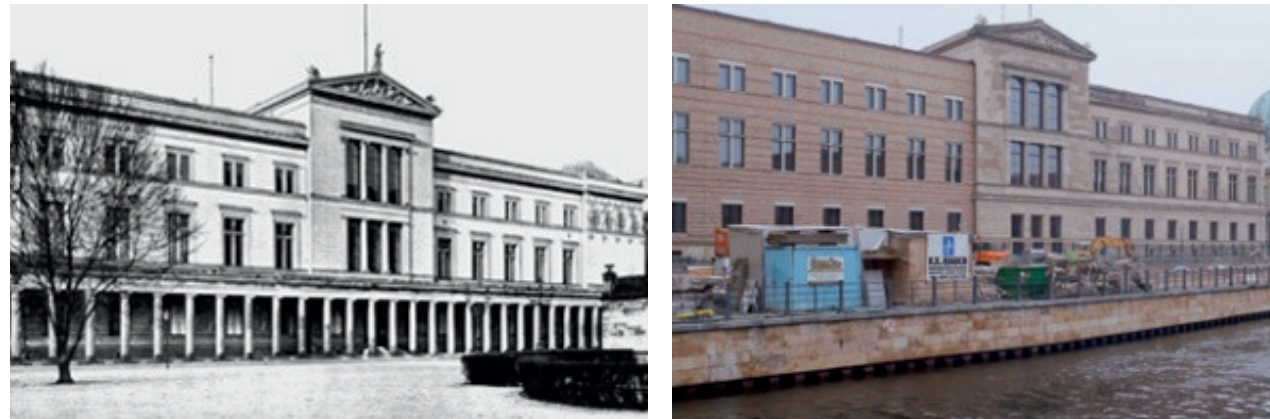
Figure 19,20 : Comparative views illustrating structural loss and its contemporary stabilisation, making absence legible through non-imitative intervention.
