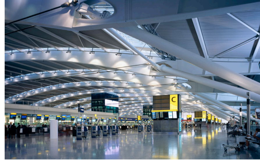
Fig. 4: Interior view of Heathrow Terminal 5 departures concourse, showing the long-span envelope and freestanding internal structures. Source: Rogers Stirk Harbour + Partners (2008).
