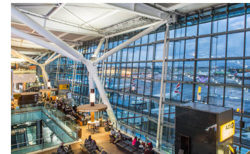
Fig. 5: Interior view of Heathrow Terminal 5 roof structure, showing the arched long-span beams supported at the perimeter. Rogers Stirk Harbour + Partners (2008).
