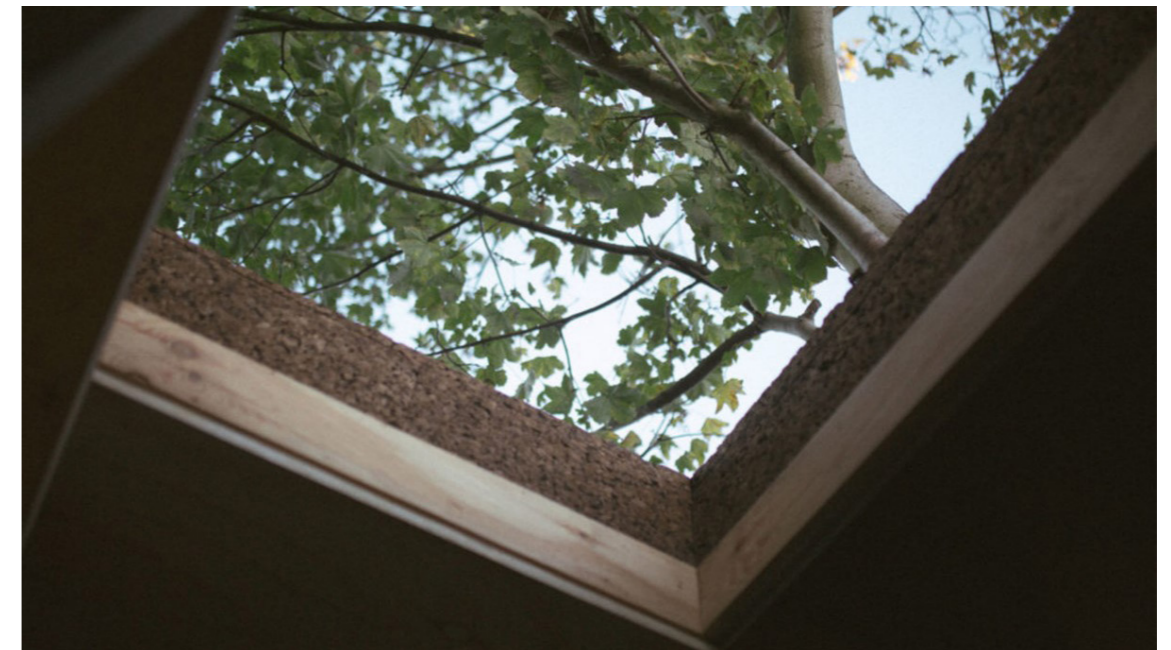
Fig.5 Opened Roof Made of Cork and Timber Joists (2018)
