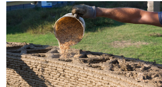
Fig.10 Waste from Rice Production Fills the Structure for Insulation (2018)
