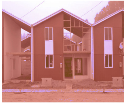
Fig. 14. 'Formal' construction stage complete, the houses are ready to be inhabited and become homes.
