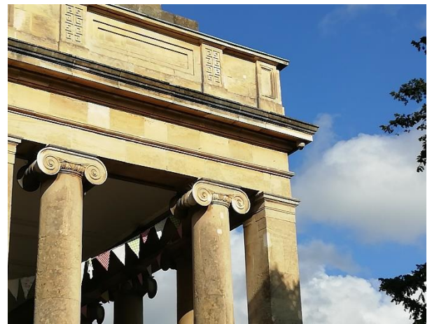
Fig. 1 Pittville Pump Room (2020)
