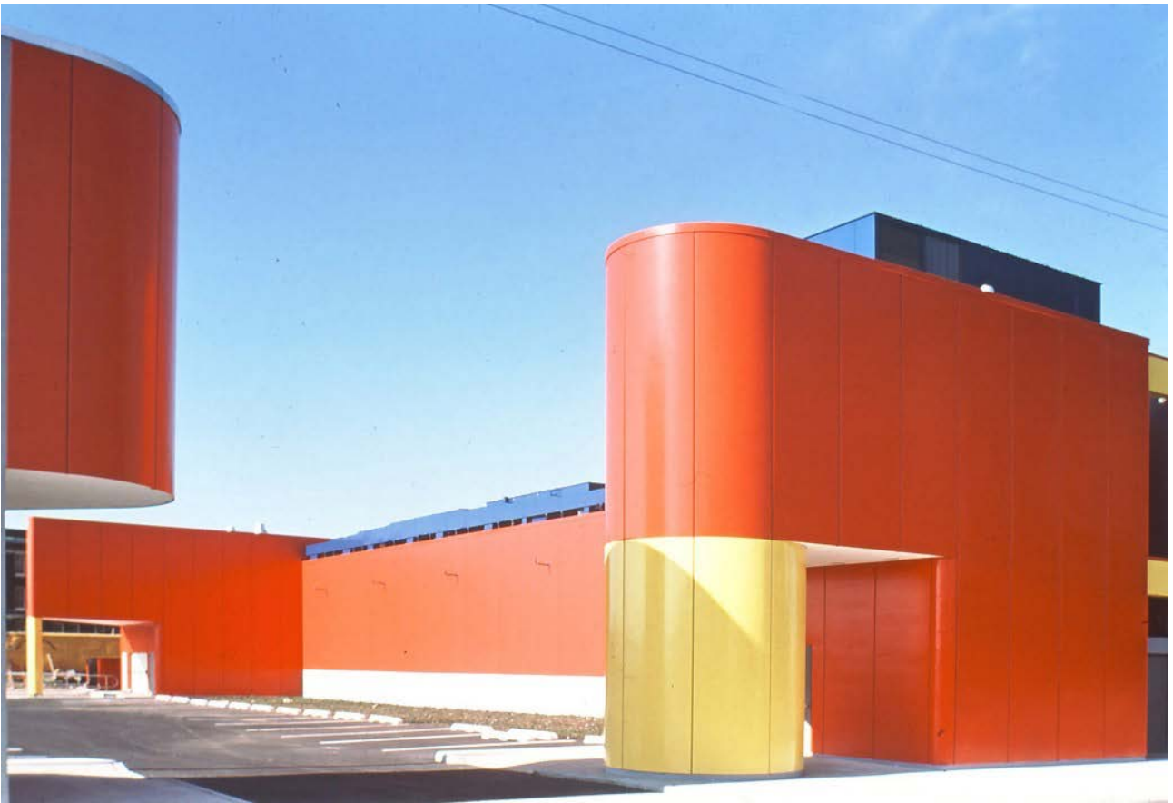
Fig. 7 Illinois Regional Library for the Blind and Physically Handicapped (1978)
