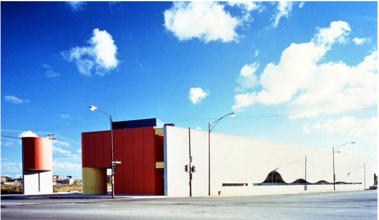
Fig. 2 Illinois Regional Library for the Blind and Physically Handicapped (1978)
