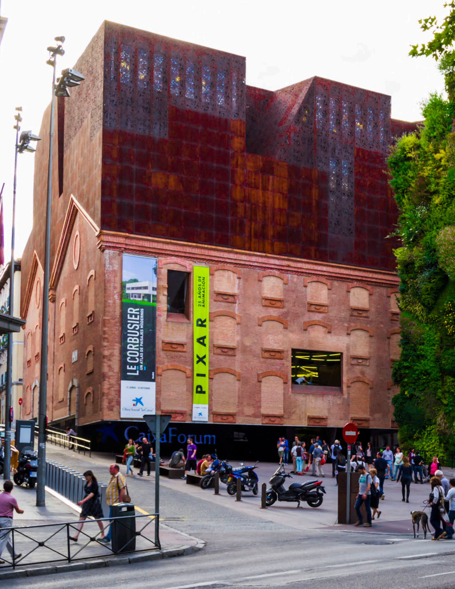
Figure 5. The exterior form of the CaixaForum Museum displaying the attached old and new structure that seemed disconnected from the ground.
