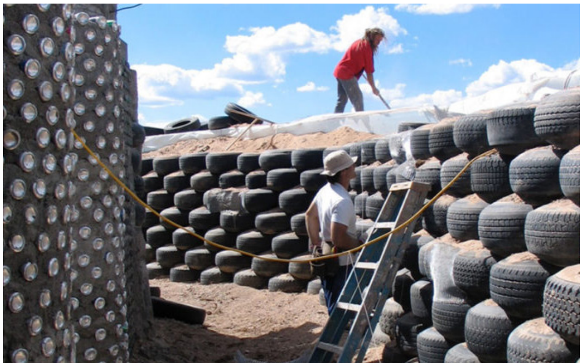
Figure 08, Construction method using recycled tyres and aluminium cans. (Earthship Biotechure, 2023)
