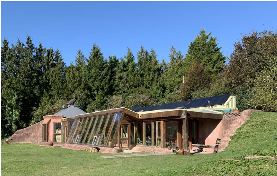
Figure 02, Photograph of Earthship in Brighton. (Taken by Millie Lawrence)
