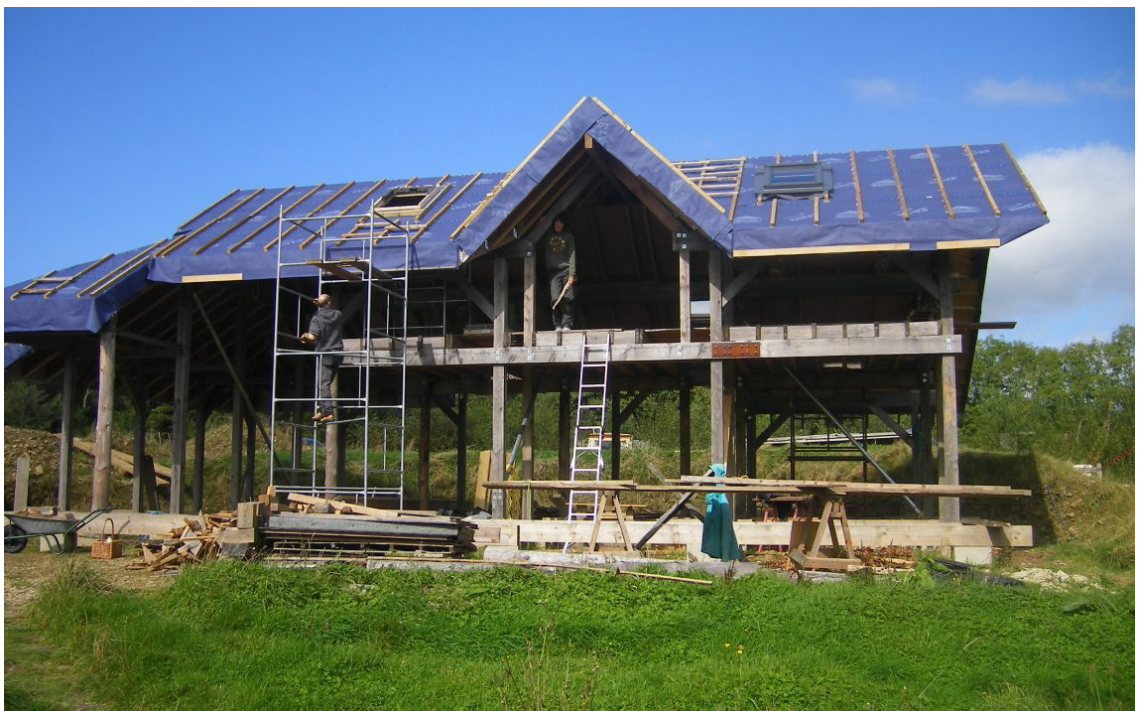
Figure 11, Timber frame house under construction. (Lammas, 2023)
