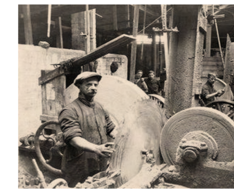
The old Grinding Shop
