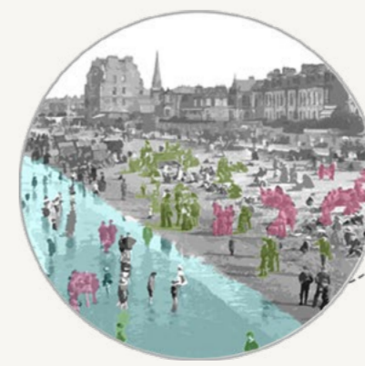
Pollution and sewage overflow
