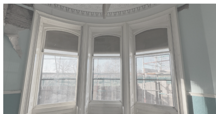
Original Wall Decoration
