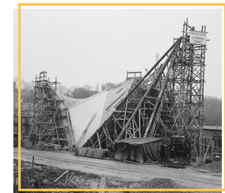
Figure 14: Philips Pavilion Construction
