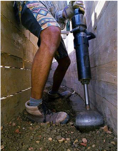
Fig. 16 Compression through mechanical trench Compactors
