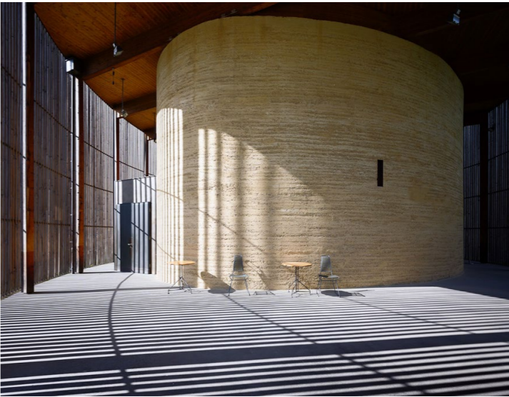
Fig. 5 Rammed Earth Body of the Chapel
