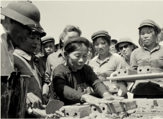
Fig 13: "Heroic mother laying the first bricks to rebuild Vinh City in collaboration with East German architecture" (Vietnam News Agency, 1972)
