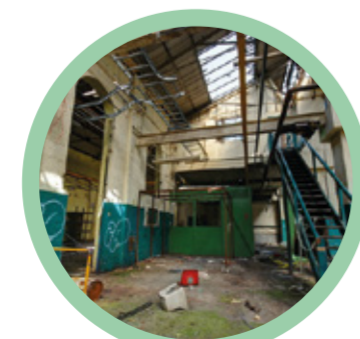
INTERIOR OF AIDA BLISS (EAST SIDE)
