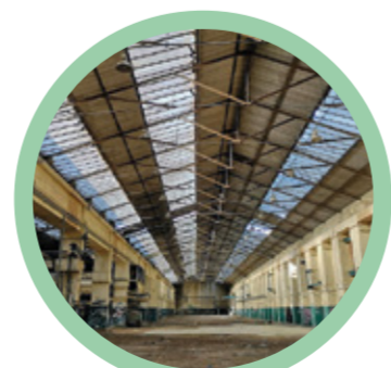
INTERIOR OF AIDA BLISS (EAST SIDE)
