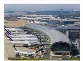
Charles De Gaulle Terminal 2E International Airport in Paris. In public buildings where the user size can change at any point the modularity is a common technic to build. The Terminal 2E was built in arched pieces which allow for the curved aesthetics to be maintained while remaining open to future additions.
