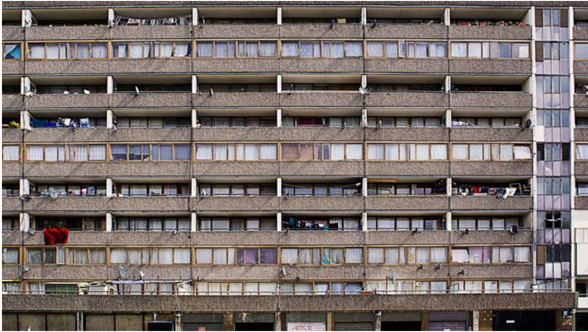
Figure 4 Exterior of the Aylesbury Estate
